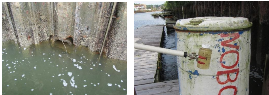
Glen Cove Creek discharges: malfunction of pump station during cleanout of the STP UV system (top, l, 7/11/18); brown discharge from north bulkhead (top, center, 7/17/18); white discharge from CSHH #10 (top, r, 10/31/18); brown discharge at CSHH #9 and water sample (bottom, 9/19/18) (photos by Carol DiPaolo)
