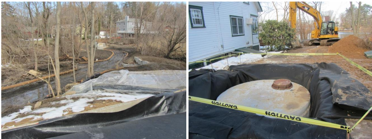
Scudder's Pond restoration and construction work: coir banks for stream from upper pond (l) and new stormwater basin for country club cottages (r) (photos by Carol DiPaolo, 3/11/14)
