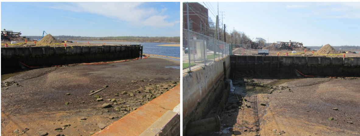
Unusually low tide at power plant demolition site; CSHH #14 is outside of the boom at the corner of the bulkhead (l) and #14A is the large outfall along the road (r)(photos by Carol DiPaolo, 4/22/15)
