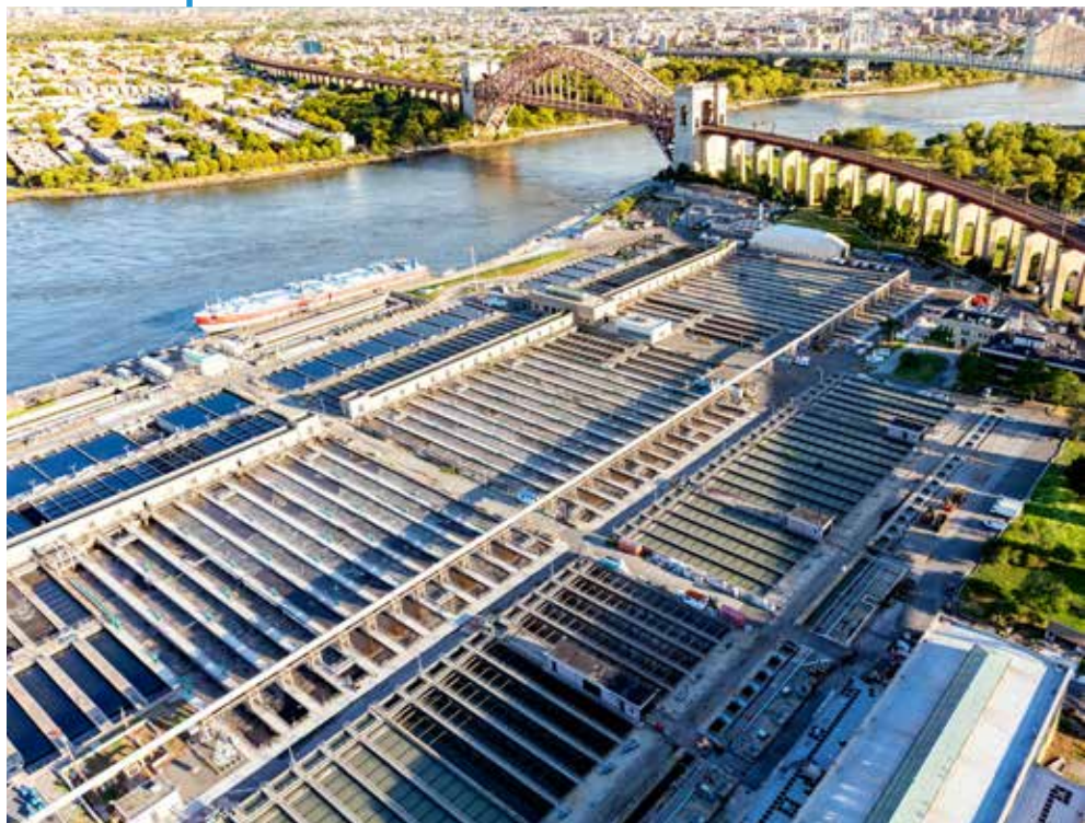
Above: Wards Island Wastewater Treatment Plant in NYC, Randall's Island
