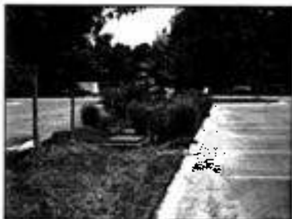
Figure 2: Parking Lot Island Turned Bioretention Area
