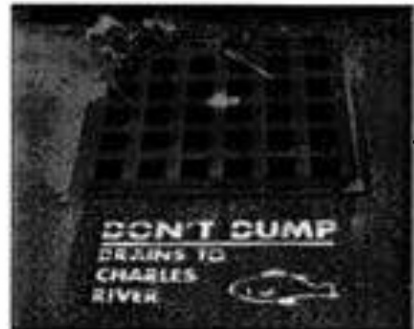
Figure 1: Storm Drain Marking
