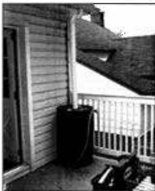
Figure 2: Rain Barrel Used on a Back, Second Floor Balcony
