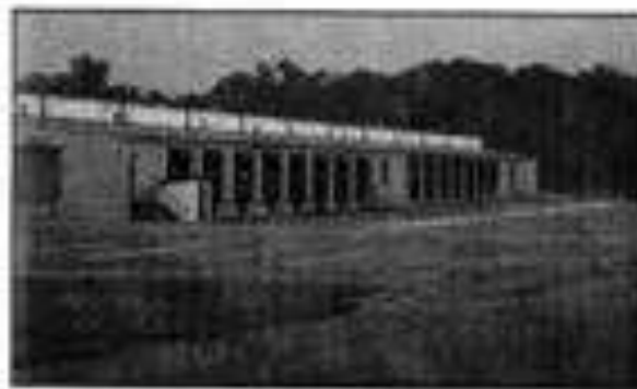
Figure 1: Loading/Unloading Area of Warehouse
