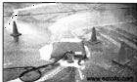
Figure 2: Storm Drain Cover Used when Washing with Soaps
