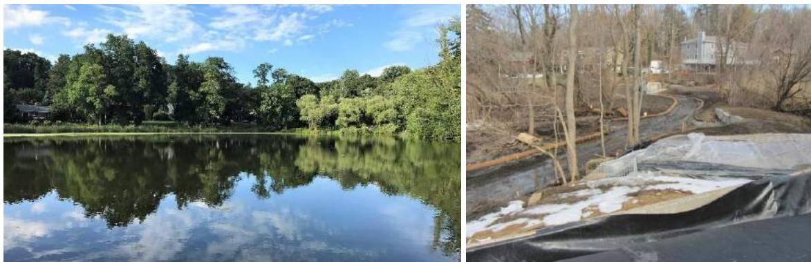
Scudder's Pond in 2020 (l) and coir banks for stream and upper-pond restoration in 2014 (r) (photos by Michelle Lapinel McAllister, 7/20/20, and Carol DiPaolo, 3/11/14, respectively)
