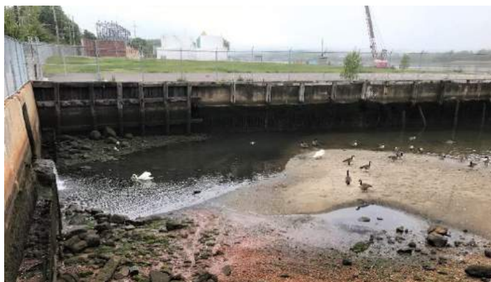
Site of the former brick powerhouse building (photo by Michelle Lapinel McAllister, 5/27/20)
