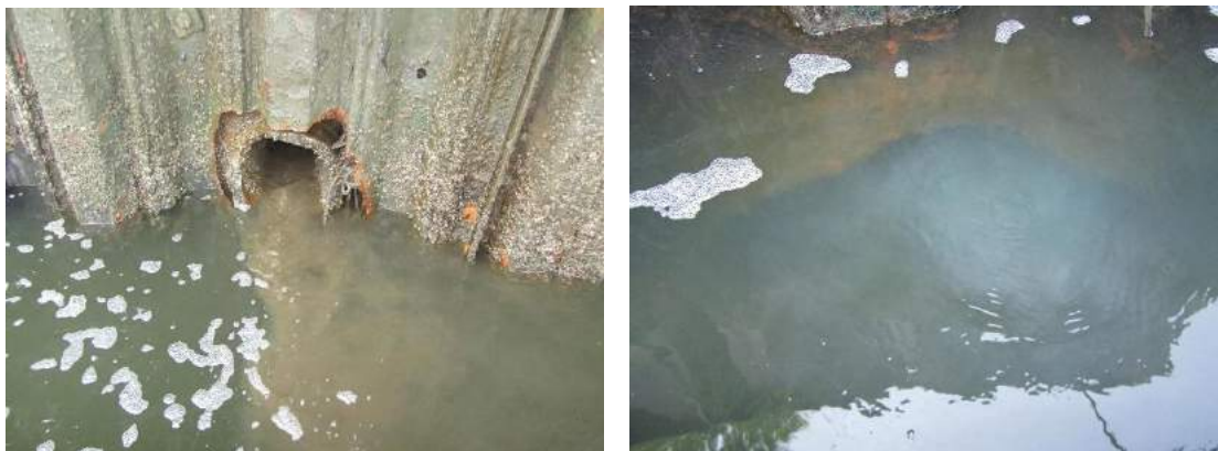
Outfalls in Glen Cove Creek: brown discharge from CSHH #9 (l); milky white discharge from CSHH #10 (r) (photos by Carol DiPaolo, 8/19/20 and 9/23/20, respectively)
