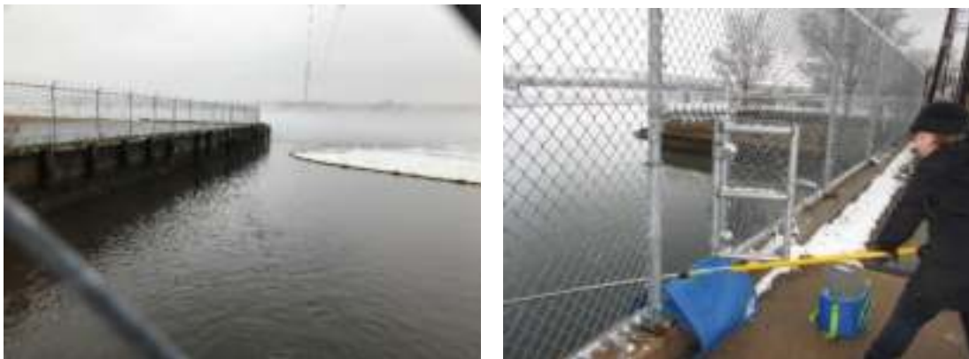
Fenced property (l) is the former site of the brick powerhouse building that was demolished in 2015 and is adjacent to outfall monitoring station CSHH #14A (r) (photos by Michelle Lapinel McAllister, 11/2/18, and Elaine Neice, 12/11/19, respectively)
