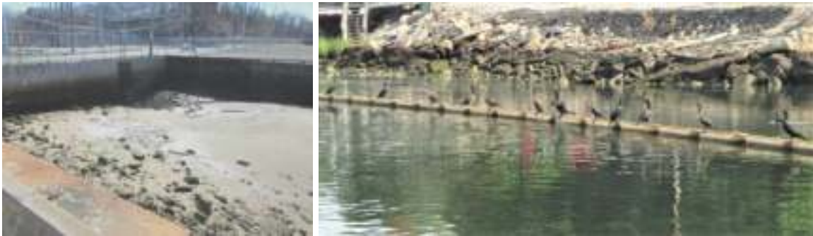
Powerhouse drain (CSHH #14A) at low tide (l) and cormorants on a boom at adjacent fuel terminal dock (r) (photos by Carol DiPaolo, 3/3/16 and 7/24/19)
