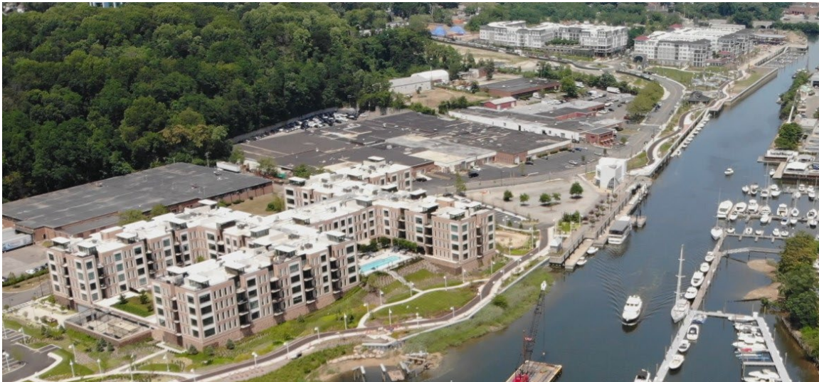
Aerial view of Garvies Point development project, Glen Cove (photo by Allen Moore, 7/21/21)
