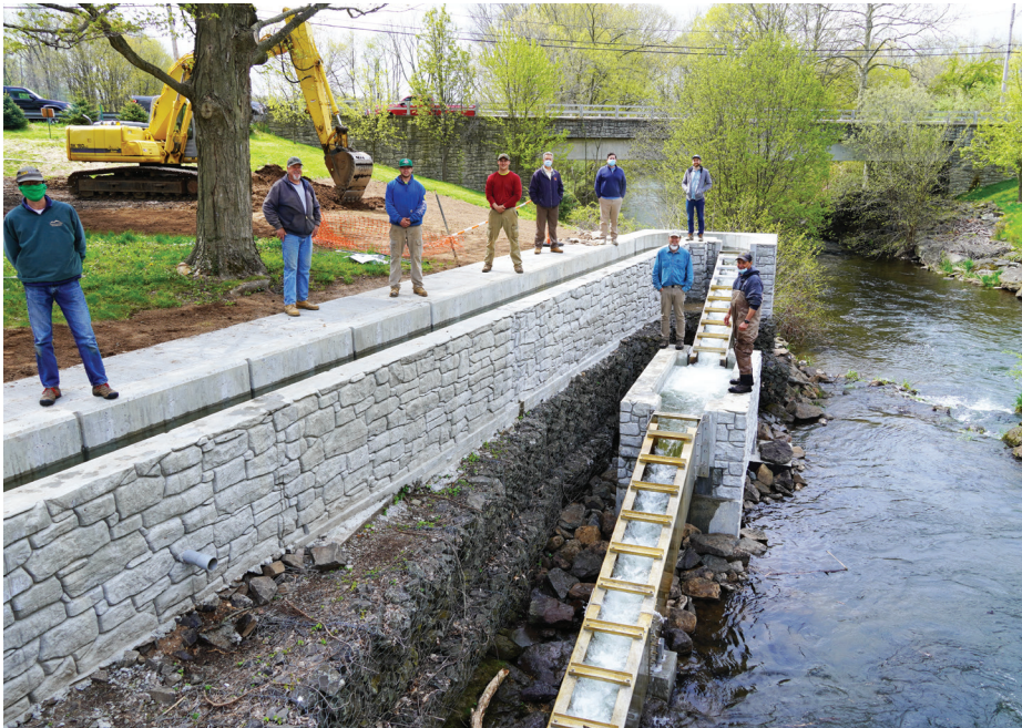
Lindsay Suter, the dam owner (foreground), surrounded by the engineering/construction team and project partners CTDEEP and Save the Sound on the Pages Millpond Dam and fishway during a project inspection in May 2020.
