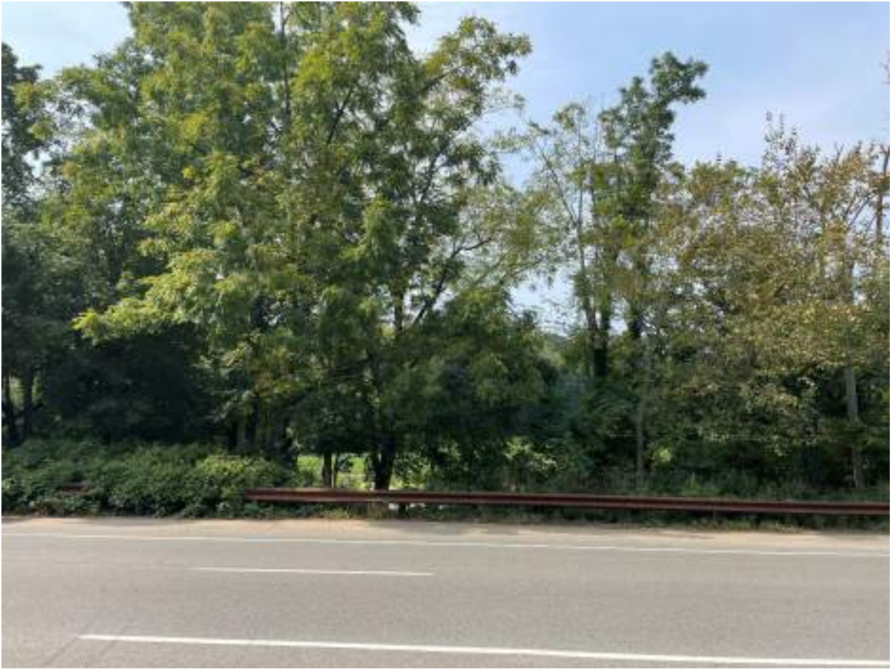
GHCC- 1: View across Cedar Swamp Road near northeast corner of Glen Head Country Club property, facing west.
