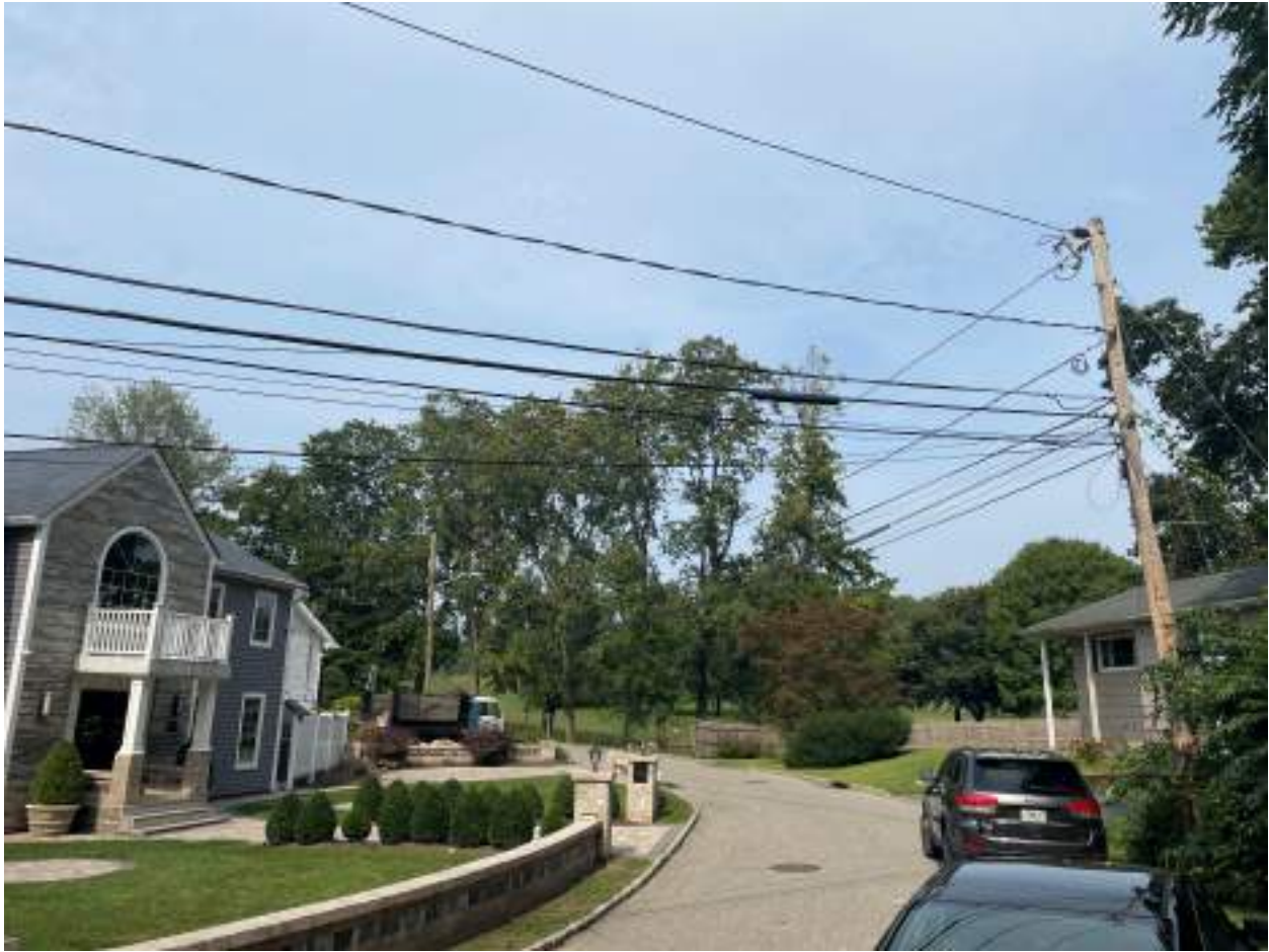
GHCC- 3: View along Hill Drive at south end of Glen Head Country Club, facing northwest.
