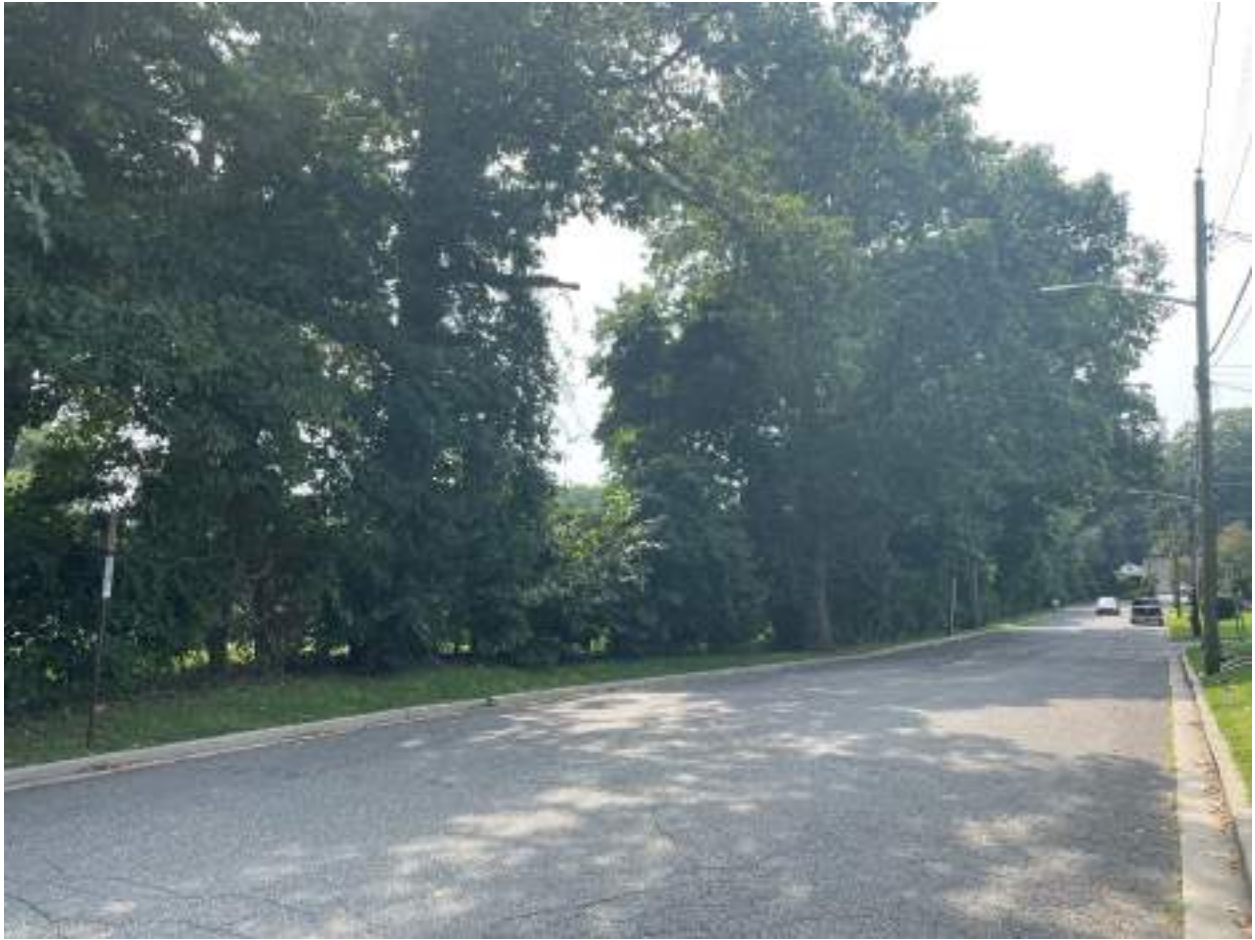
NCC- 1: View along Nassau Road near northwest corner of Nassau Country Club property, facing southeast.
