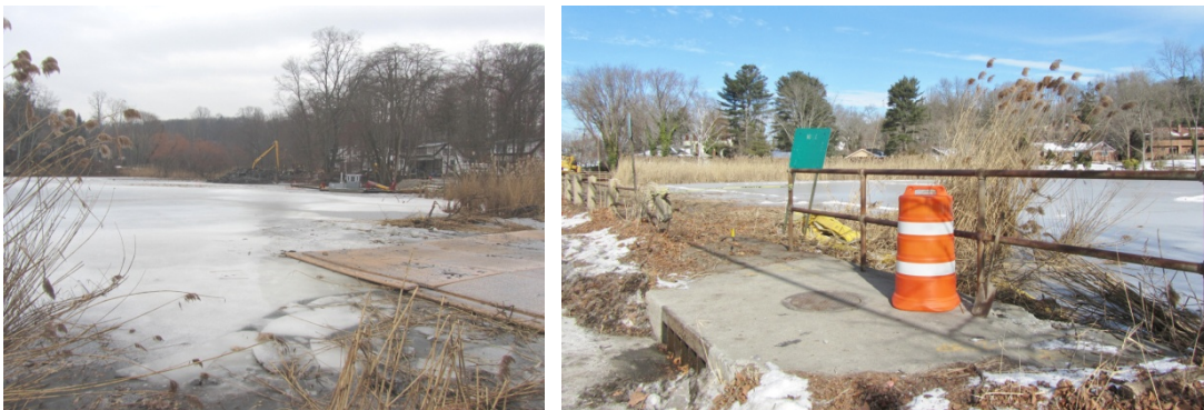
Freezing temperatures caused a delay in dredging Scudder's Pond (l) and in phragmites removal near the weir (CSHH #15B) (photos by Carol DiPaolo, 1/28/14)
