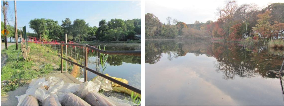
CSHH #15A during placement of coir tubes for new plantings at Scudder's Pond (l) and an autumn view of the pond postconstruction (r) (photos by Carol DiPaolo, 7/2/14 and 10/29/14, respectively)
