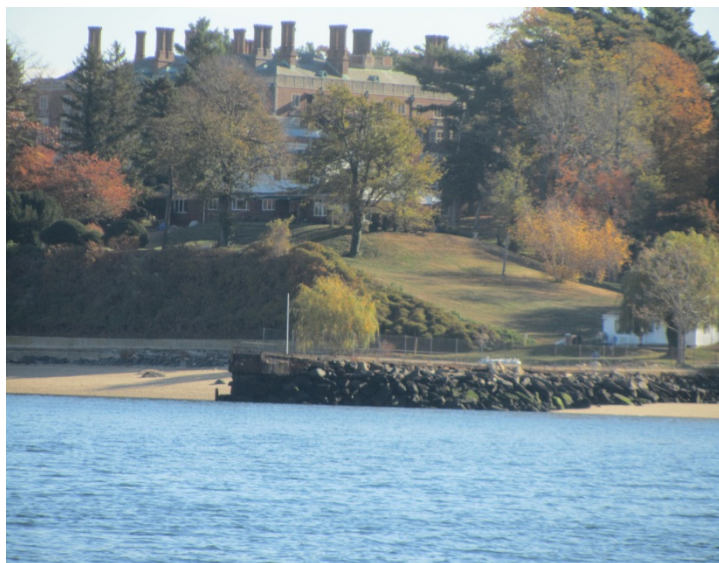
Webb Institute on the east shore of Hempstead Harbor (photo by Carol DiPaolo, 11/6/13)
