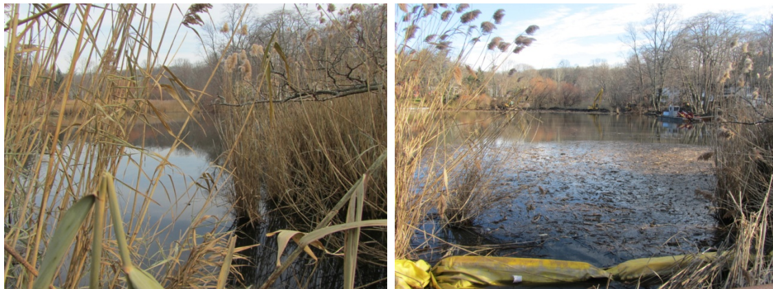
Scudder's Pond prior to construction work (12/3/13) and after start of phragmites removal (12/24/13) (photos by Carol DiPaolo)
