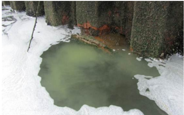
White flow from pipe at CSHH #10, Glen Cove Creek (photo by Carol DiPaolo, 6/8/11)
