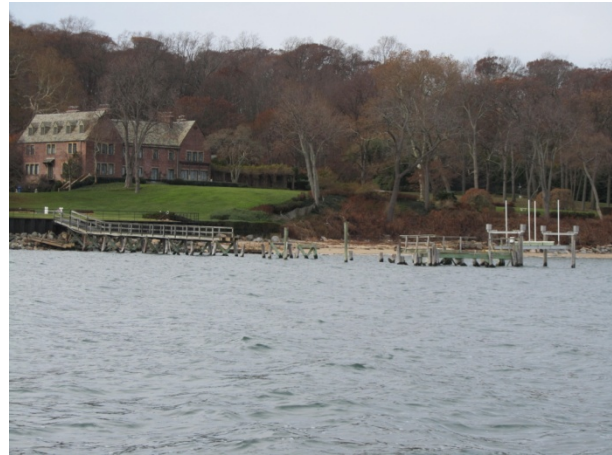
Dock damage on the western shore of the harbor following Superstorm Sandy (photos by Carol DiPaolo, 11/16/12)
