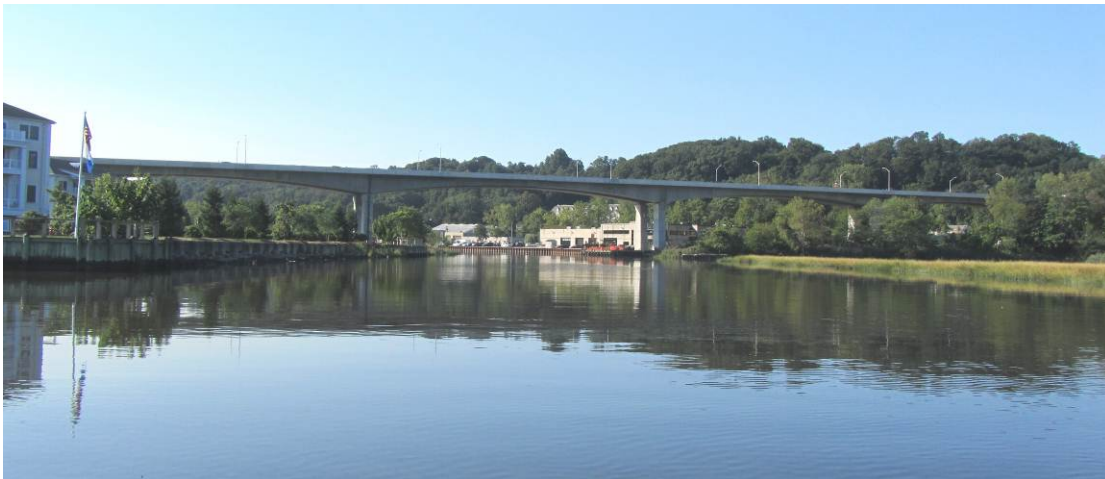
The new Roslyn viaduct renamed to honor William Cullen Bryant, the prominent 19 th century poet and journalist who resided at the Cedarmere Estate on the eastern shore of Hempstead Harbor (photo by Carol DiPaolo, 9/12/12)
