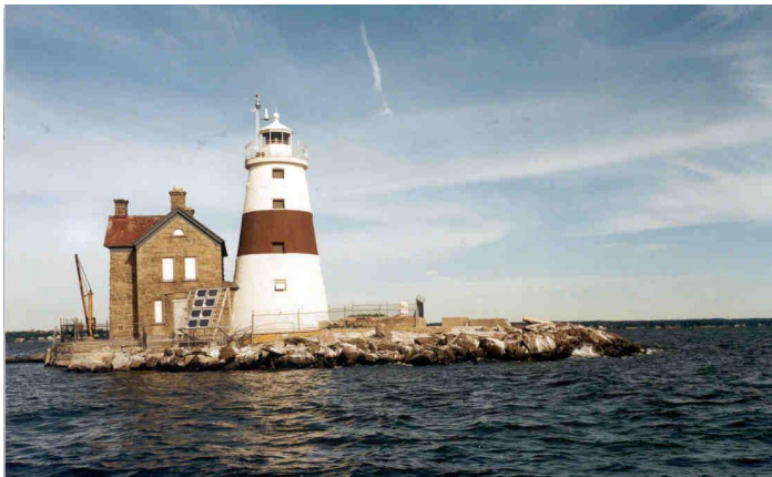
Execution Lighthouse, 2005 (Photo: Carol DiPaolo)
